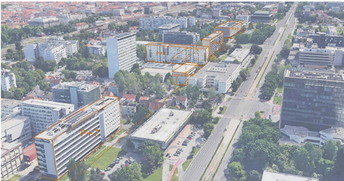
Figure 2. Second row of buildings in Vukovarska Street
